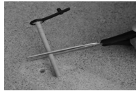
Cut sleeve according to measuring depth
